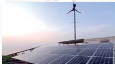
New Energy Lab, Public Authority for Applied Education & Training (PAAET), Kuwait, page 15
